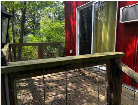
Utility Shed Deck
